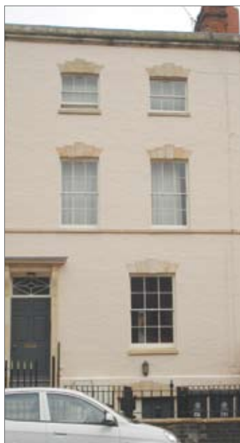
131 Southgate Street after
