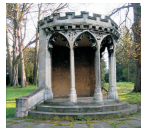
King's Board, Hillfield Gardens, London Road Late 18th century gazebo, incorporating a re-used 14th century arcade and other architectural details said to come from the King's Board, a medieval house which stood in the city centre until demolition in 1780, Grade II*.
