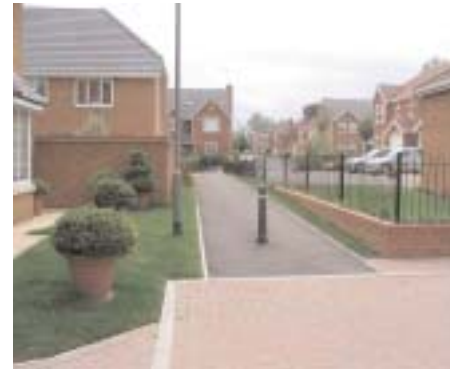
A user-friendly, well-lit footpath link with houses overlooking it and clear views through.
