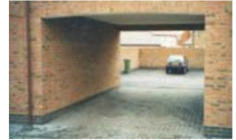
This parking court does not benefit from internal natural surveillance and the entrance is poorly defined. This clearly has the feeling of a parking area rather than a place in its own right. The paving is the same as that in the public area. This reduces the feeling of this being a private space and will not be as effective in deterring people who have no purpose in entering.
