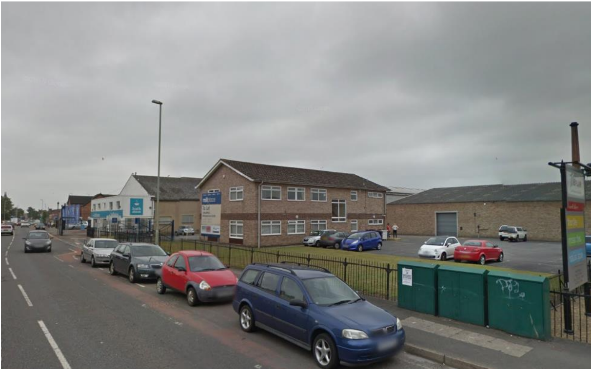
Plate 1 Northern part of HA21 site from the north east
