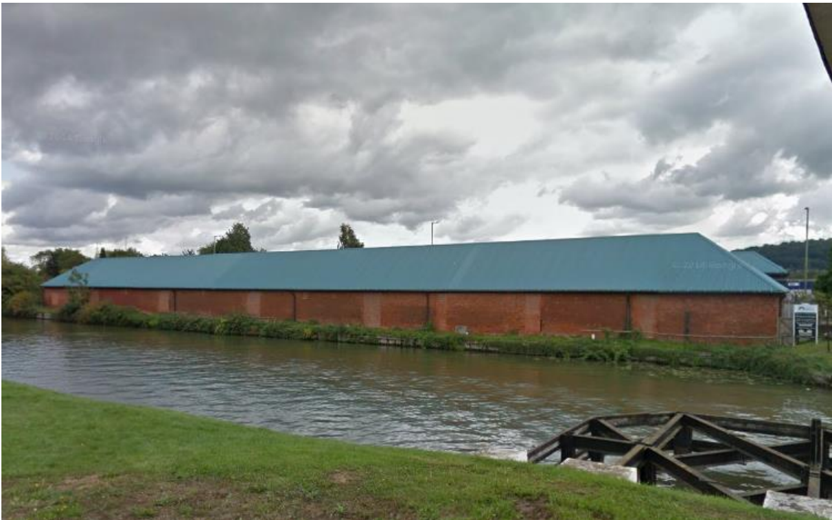
Plate 3 The southern salt warehouse on Bristol Road, from the west
