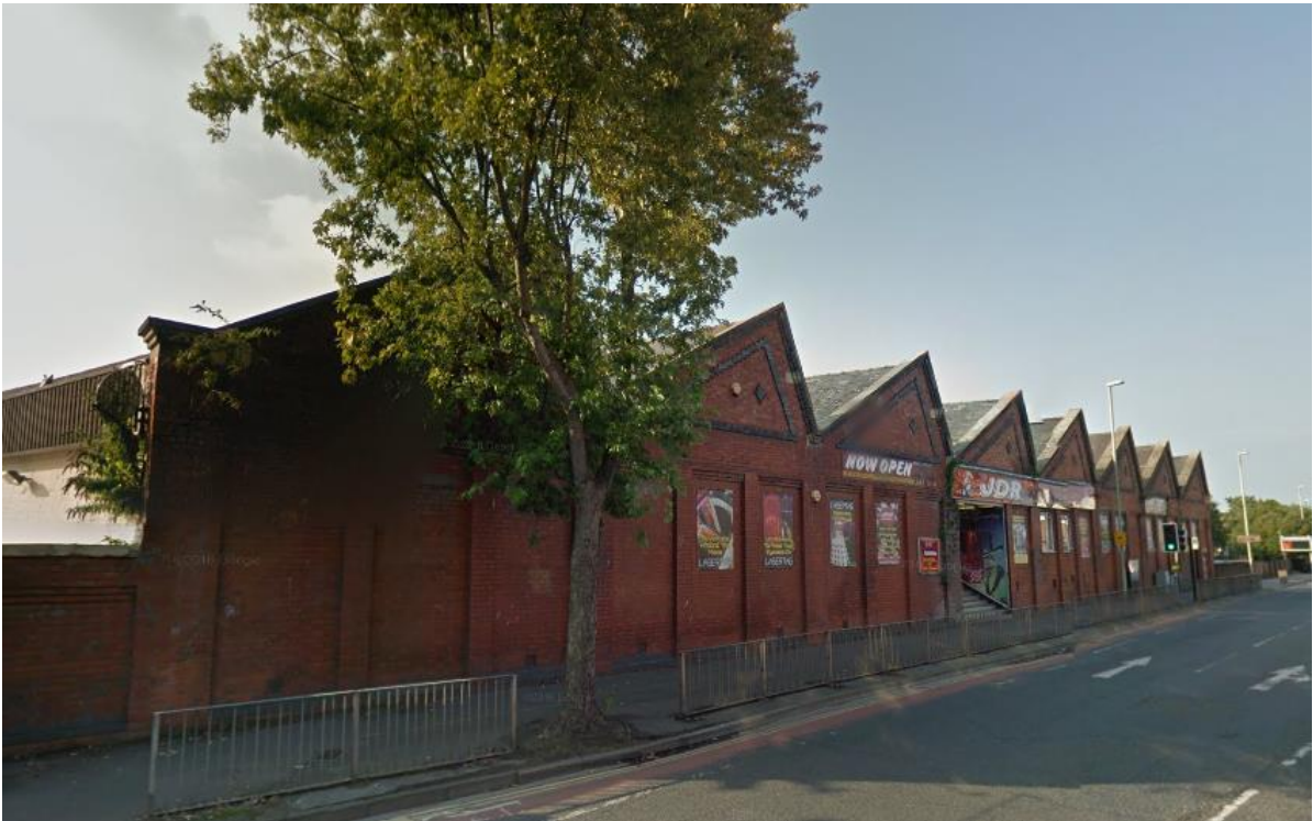
Plate 6 Last surviving building of the Gloucester Railway Carriage and Wagon Works
