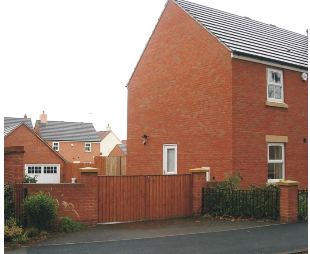
In this development boundary walls at the side of properties, which do not interfere with the potential for maximising natural surveillance, have been constructed to a height which screens the wheelie bin. The addition of these lockable gates provides extra security, and solidity to the build line.
