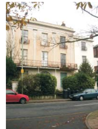
In this example the hedge used to define the public and private space has not been maintained at a low level and now obscures the sight lines between the house and the street. This ultimately reduces the opportunities for natural surveillance, increase the fear of crime and the opportunities for crime.
