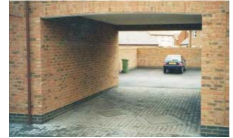
This parking court does not benefit from internal natural surveillance and the entrance is poorly defined. This clearly has the feeling of a parking area rather than a place in its own right. The paving is the same as that in the public area. This reduces the feeling of this being a private space and will not be as effective in deterring people who have no purpose in entering.
