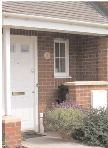
Well designed and integrated bin storage.
