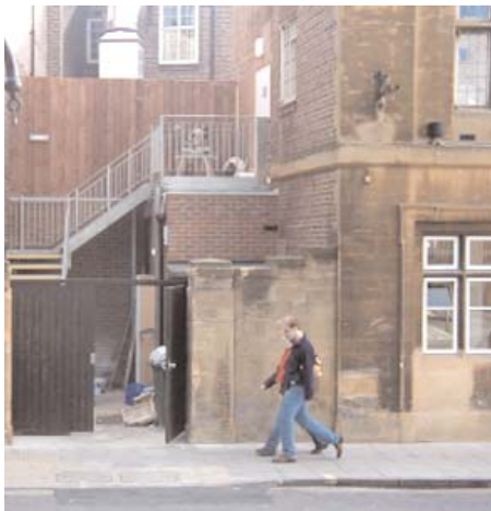
These gates have been used to conceal a bin storage area and provide security to an external staircase however they have not been properly managed or maintained and there is a limited sense of ownership. They are consequently left open creating an unattractive streetscape and compromising security.
