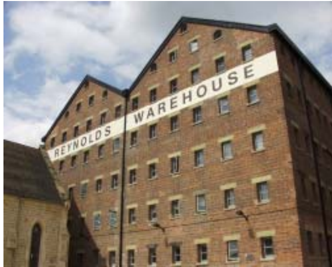
Photo 2 - Double Reynolds Warehouse
