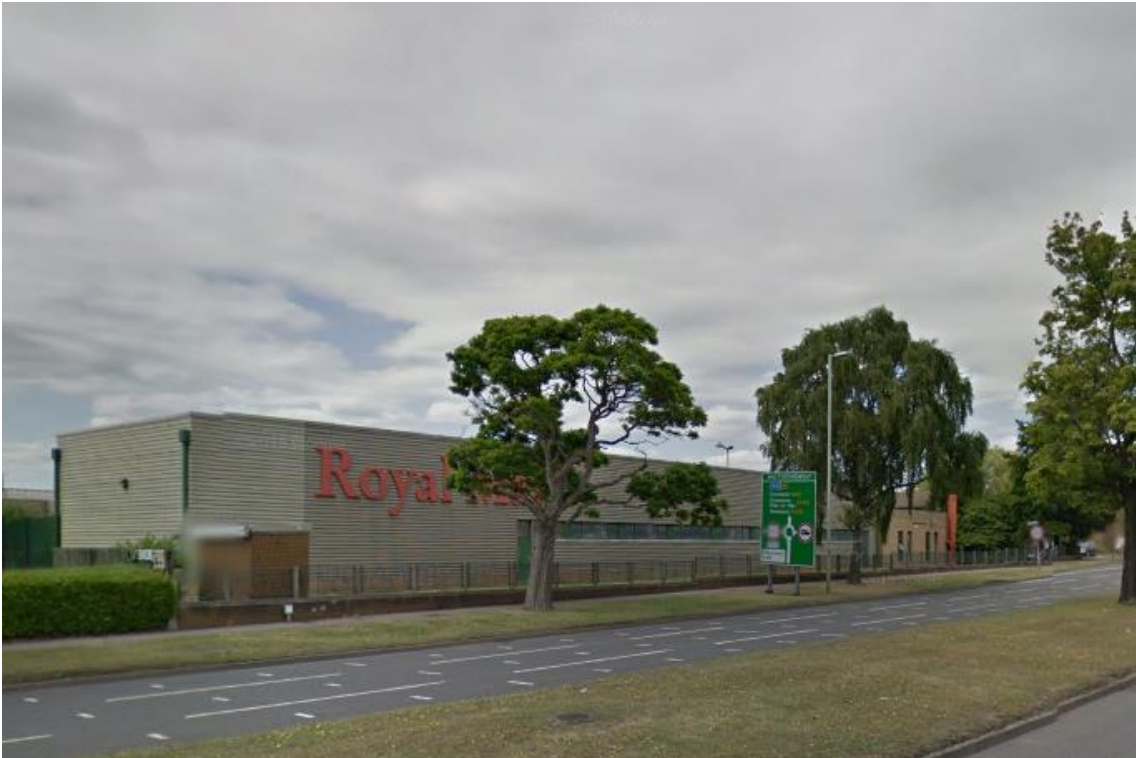
Plate 1: The FS05 site from the south east
