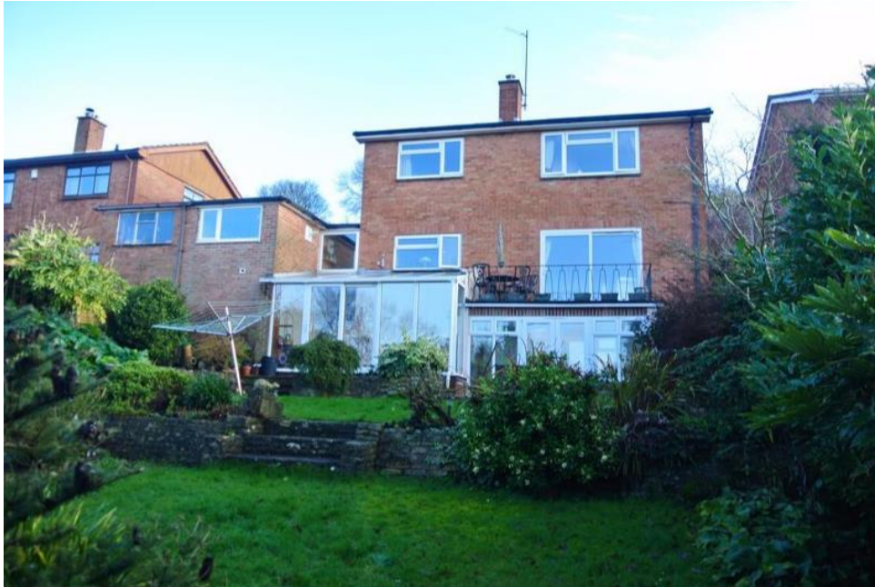
First floor raised terrace above lower ground floor extension at no. 7 Ardmore Close
