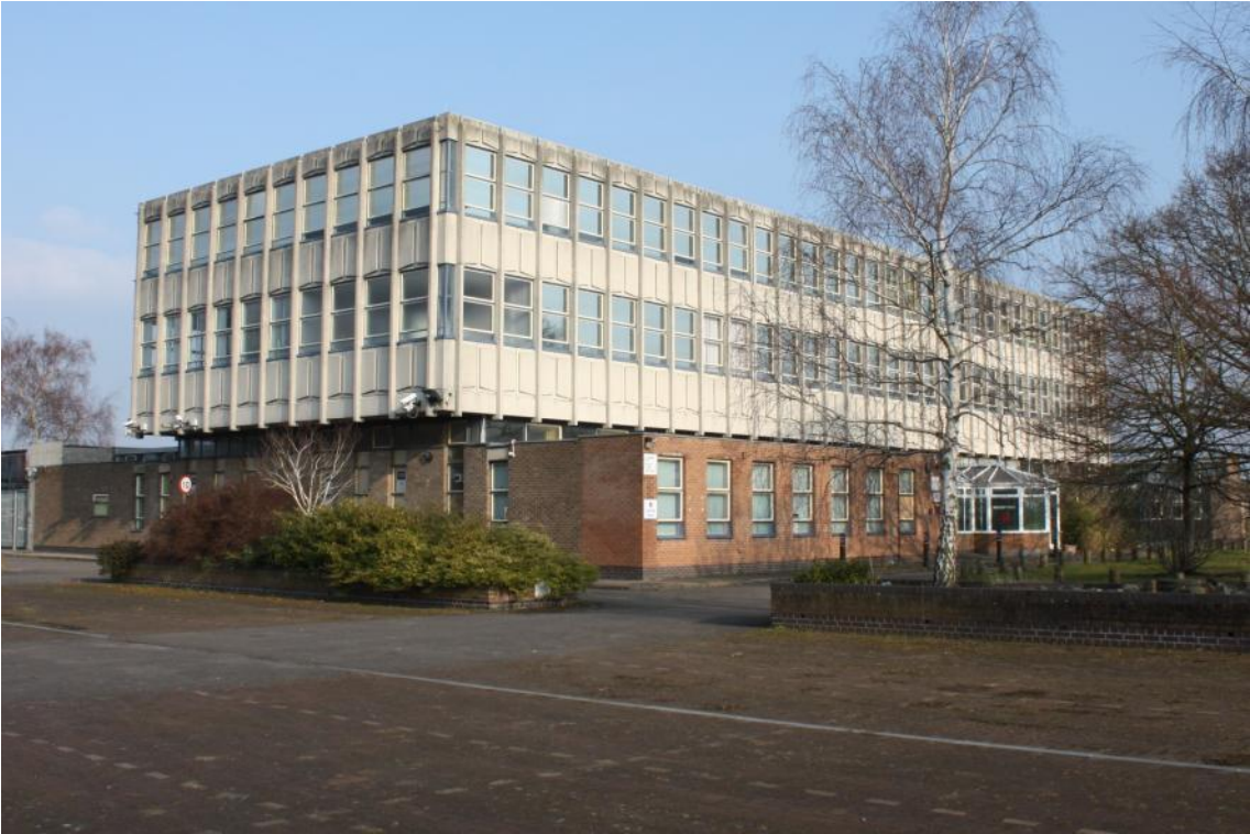
Plate 3: View of main school building from the south east
