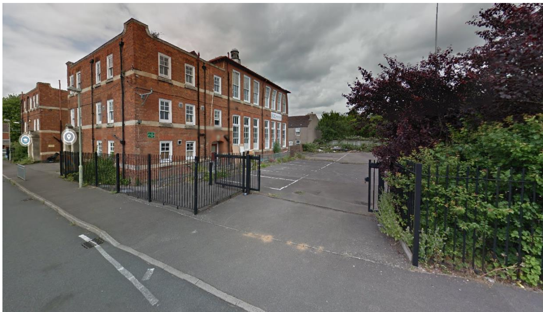
Existing access from Colwell School Close
