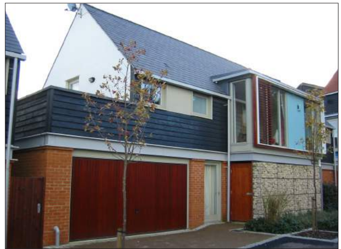
Fig 5.16: Integral garage positively designed into façade with habitable rooms providing ground floor overlooking to the street and an active frontage.
