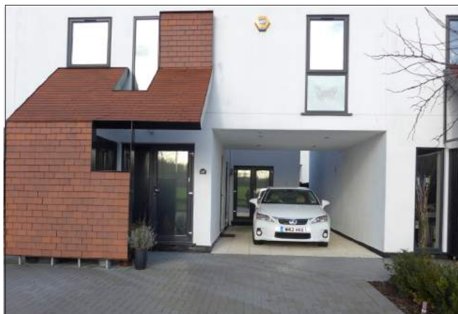
Fig 5.15: Wide frontage, shallow depth unit types allow parking to be tucked under the building
