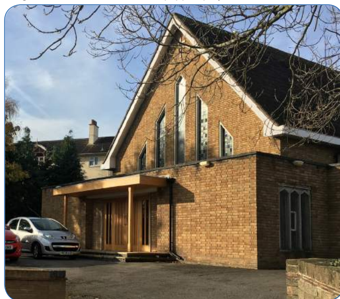
Fig 2.7: Example of existing community facilities in Matson: St Augustines Church
