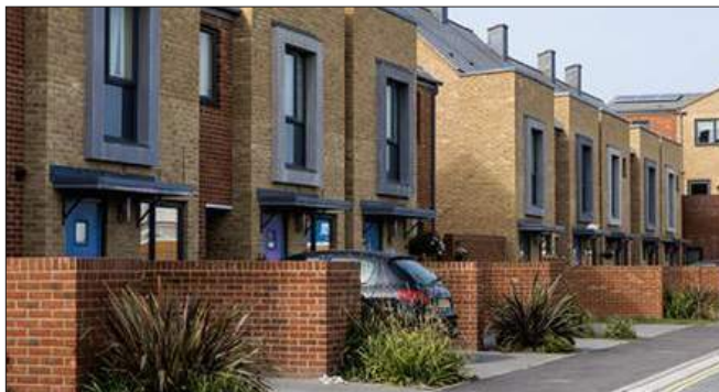
Fig 5.14: A combination of brick walls and soft landscape used to reduce the visual impact of cars and create clearly defined front garden areas.
