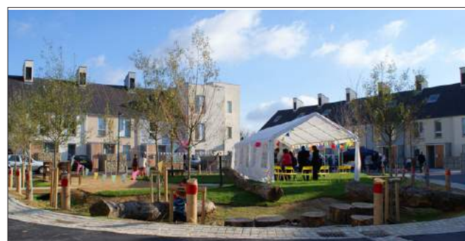
Fig 5.9: Buildings and space working together to create an attractive outlook for the new homes and a safe place to be
