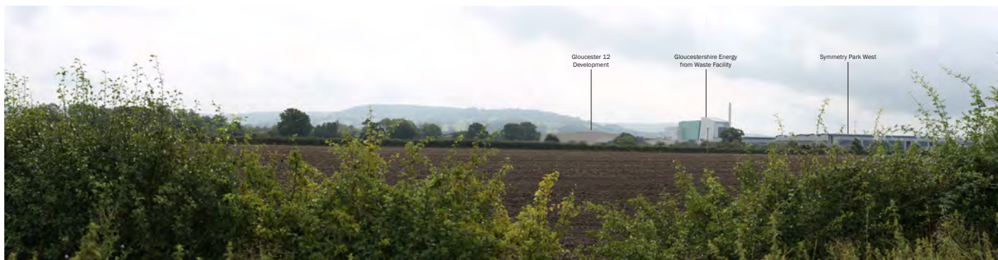
View from public footpath (Ref EHD/7/1) looking south-west - Photomontage of Gloucestershire Energy from Waste, St Modwen Park and Gloucester 12 and Symmetry Park West and East
