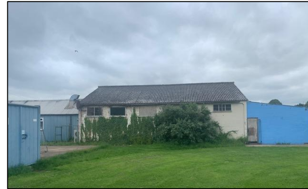
Figure 6.1 – Existing Asbestos Roof
