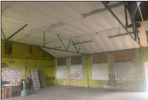
Figure 6.2 – Existing Function Hall
