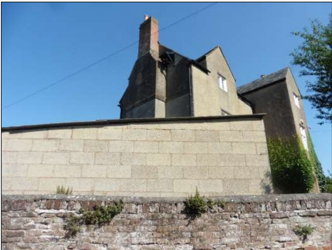
Plate 8: Breeze block garage to south of Hempsted House.
