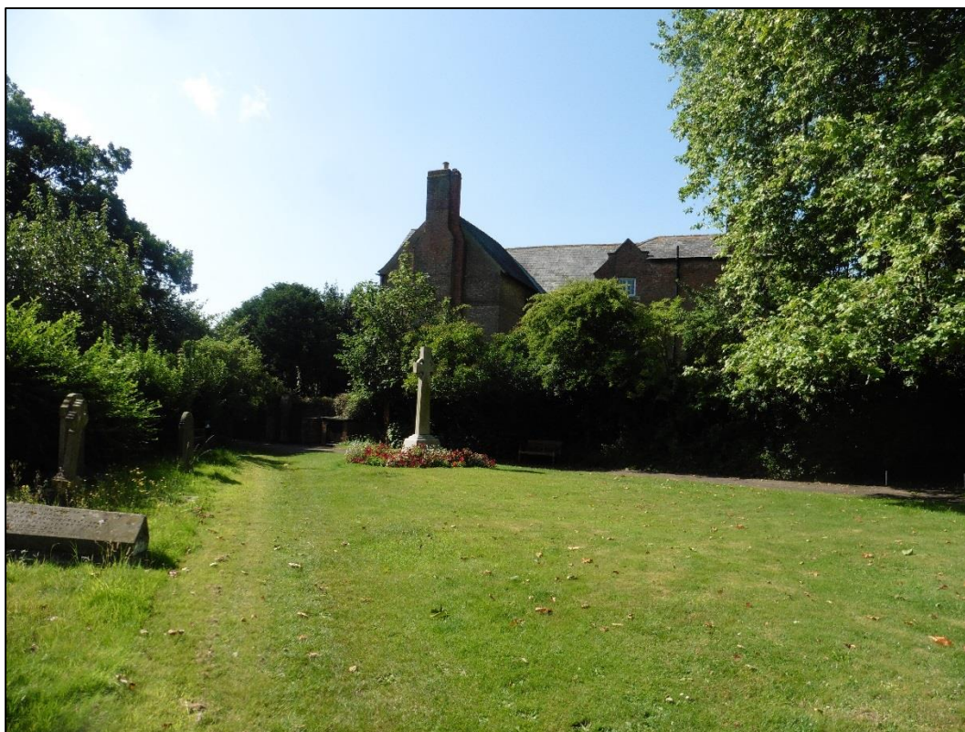
Plate 9: View south from the churchyard of St Swithun's Church of the northern elevation of Hempsted House.
