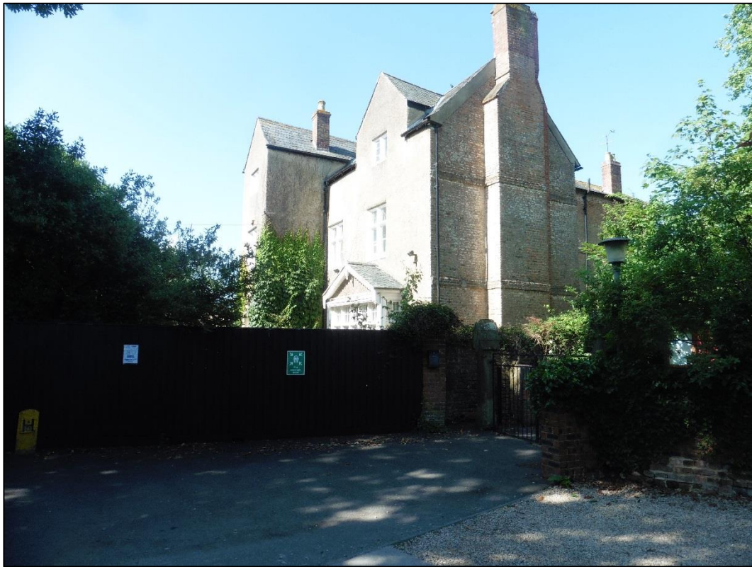
Plate 7: Hempsted House, viewed from the north-east.
