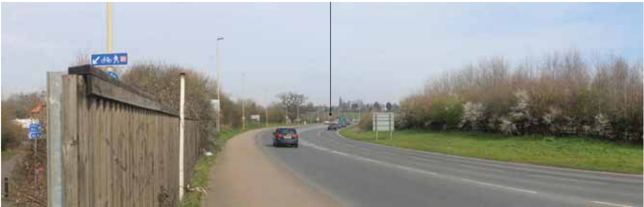
t 13 View from A430, looking north towards Site.
