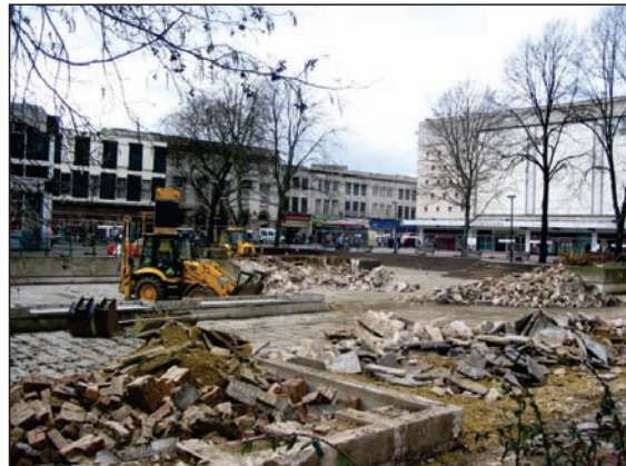
Fountains being demolished early 2006
