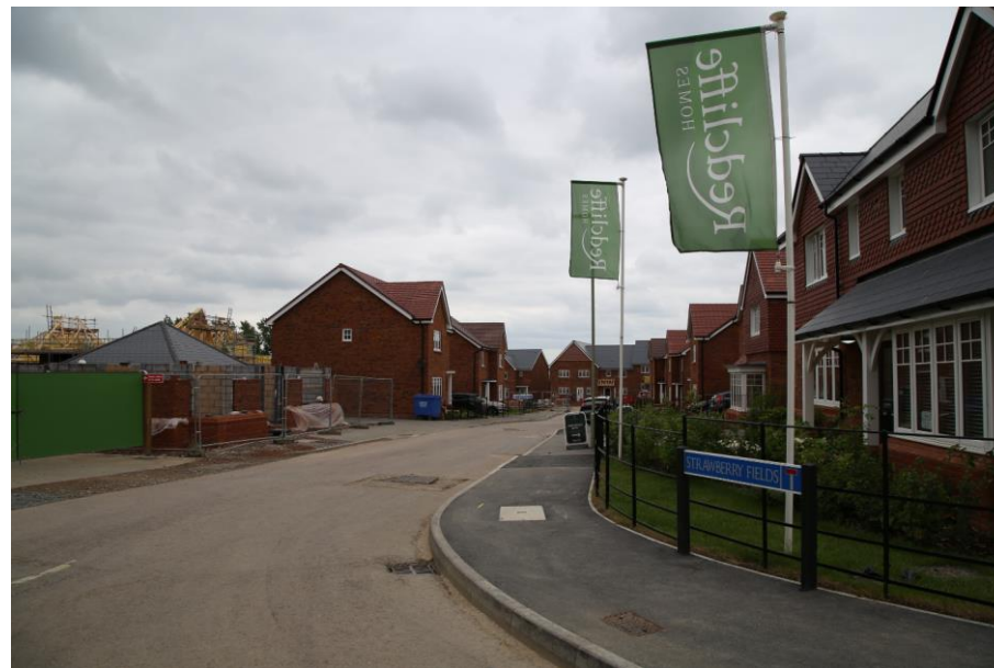
Plate 11 – Entrance to ongoing Strawberry Fields development set at the top of Rea Lane in Hempsted.
