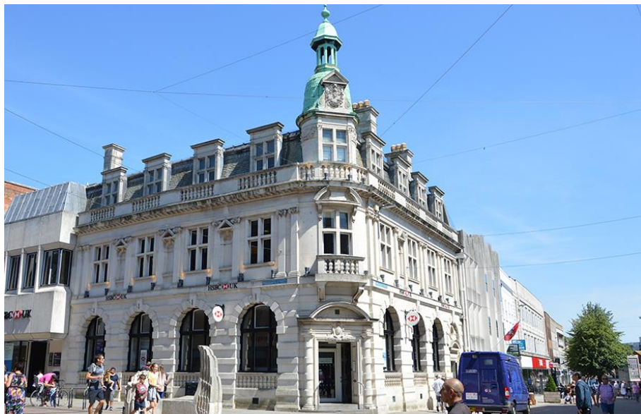
HSBC Bank, built for London, City and Midland Bank, Northgate Street – 1905-7
