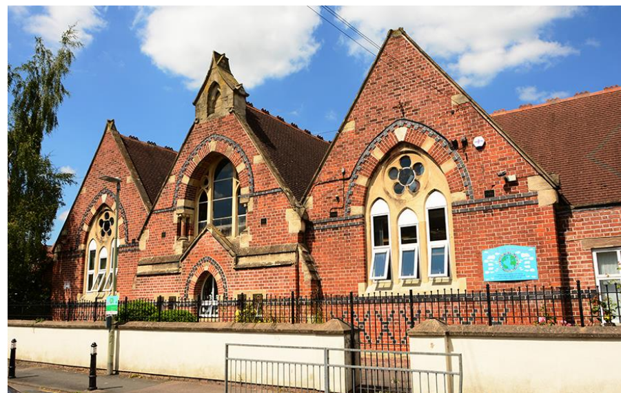
St Paul's School, New Street – Gothic Revival Church School of 1869-70
