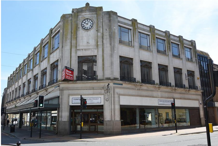
Former Co-Op stores, Easgate Street – 1929-31
