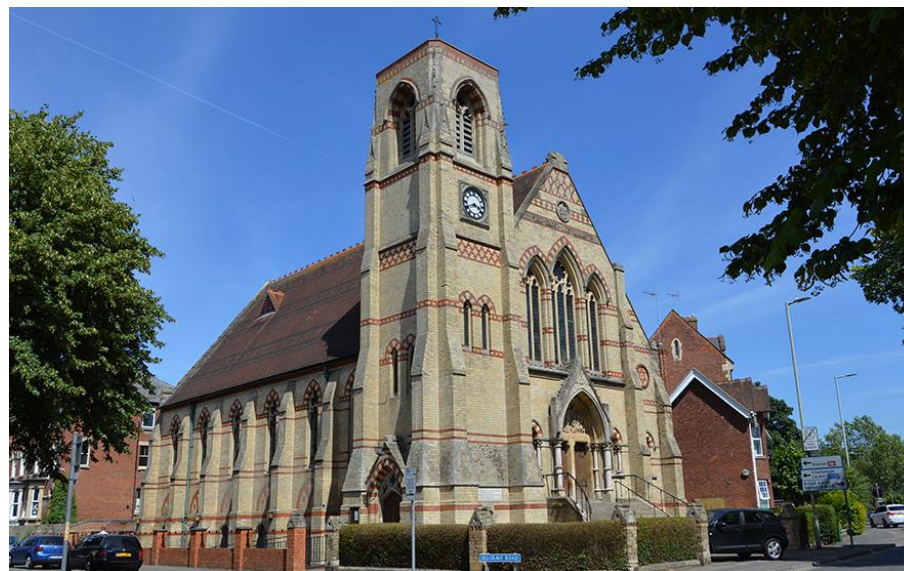
Gloucester United Reform Church, former Whitefield Presbyterian Church, Park Road – 1870-2
