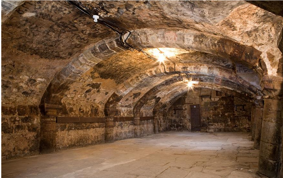
Fleece Hotel undercroft (photo supplied by Marketing Gloucester)
