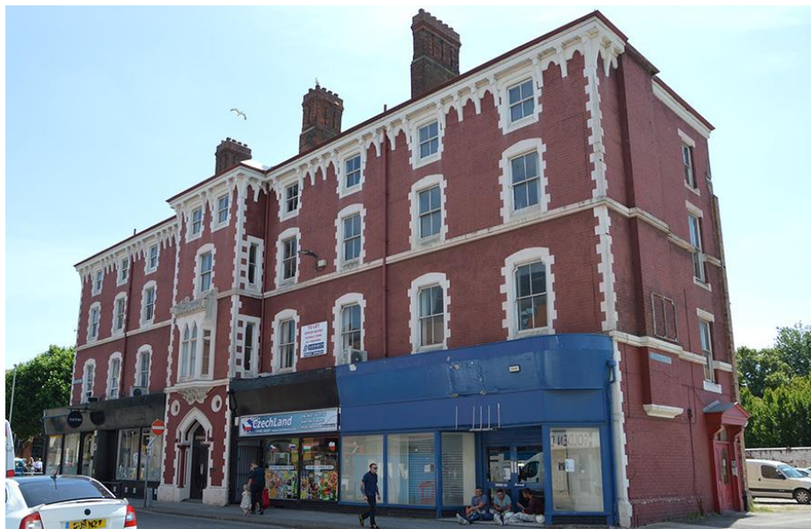
Spread Eagle Hotel, Northgate Street – 1864-6
