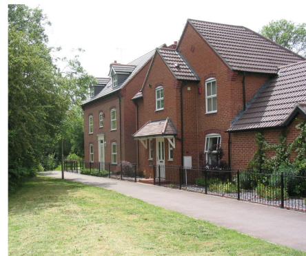
Well defined boundaries between public and private space, a well-lit surfaced route and simple planting.
