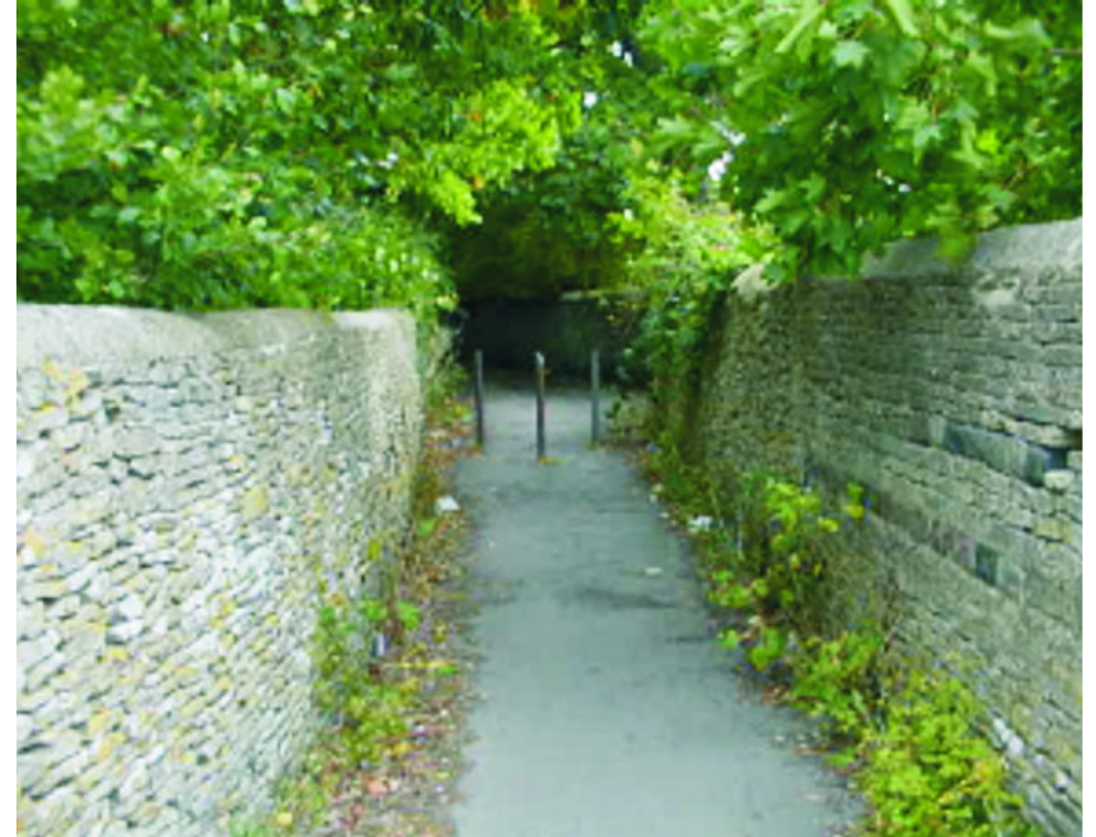
This footpath has no natural surveillance or lighting and is very narrow and enclosed by the solid walls and the overgrown planting. It is also not possible to see where the route leads. This route creates opportunities for crime and anti social behaviour and is likely to increase the perceived fear of crime by its design to those who choose to use it.
