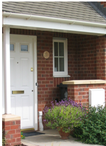
Well designed and integrated bin storage.
