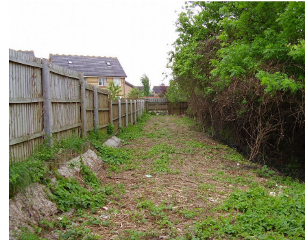
Lack of thought for watercourse access and maintenance requirements can create neglected strips of land.
