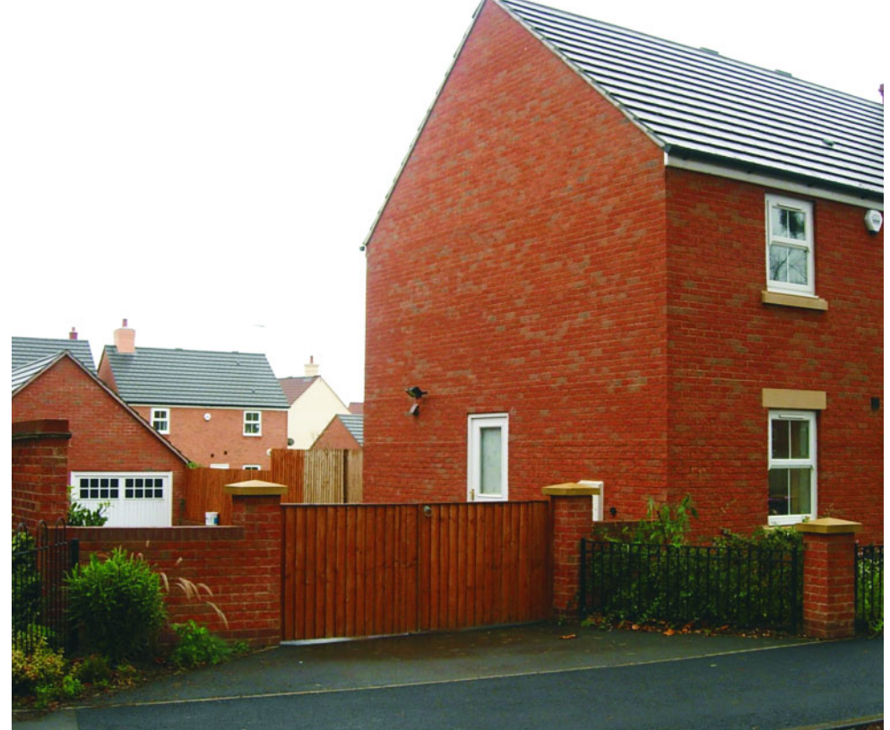
In this development boundary walls at the side of properties, which do not interfere with the potential for maximising natural surveillance, have been constructed to a height which screens the wheelie bin. The addition of these lockable gates provides extra security, and solidity to the build line.
