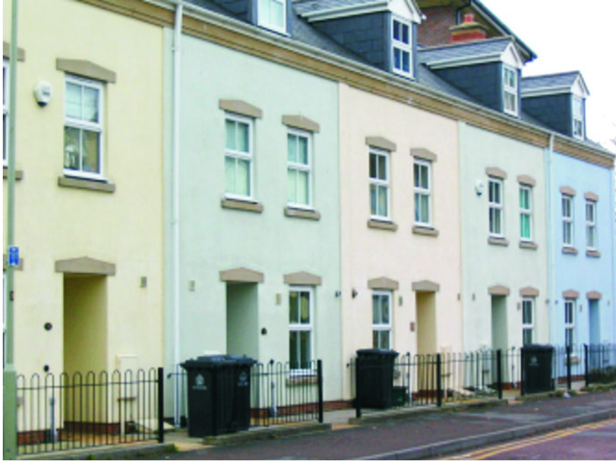
In this development adequate thought was not given to bin storage. As a consequence the bins permanently clutter the streetscene.
