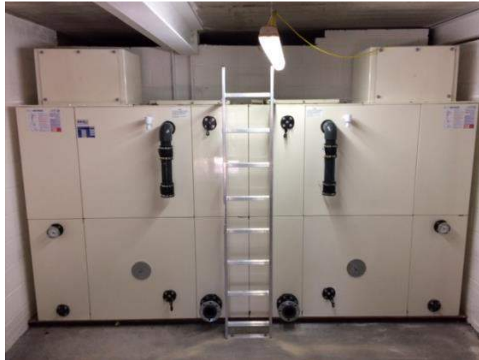
Totally Internally Flanged Tank (TIF)
