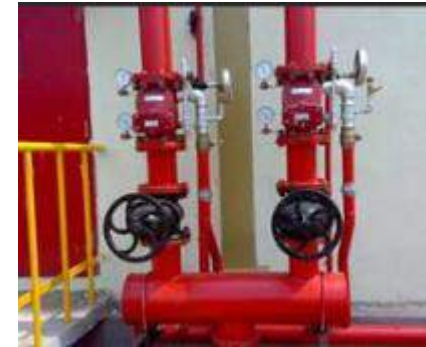
TYPICAL VALVE SET ARRANGEMENT
