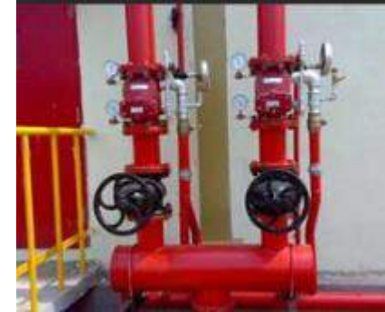
TYPICAL VALVE SET ARRANGEMENT
