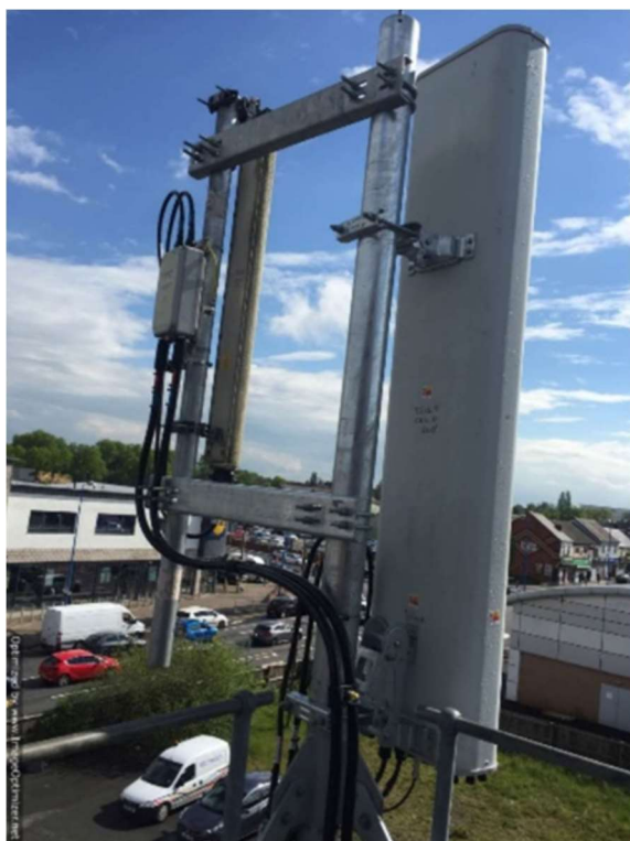
Source: Cellnex Blackheath Telephone Exchange – roof edge 5G antenna configuration
