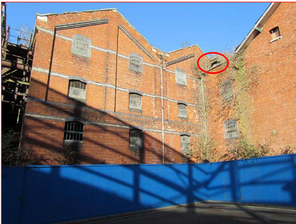
Fig.19 Downings Malthouse eastern elevation with displaced hoist circled
