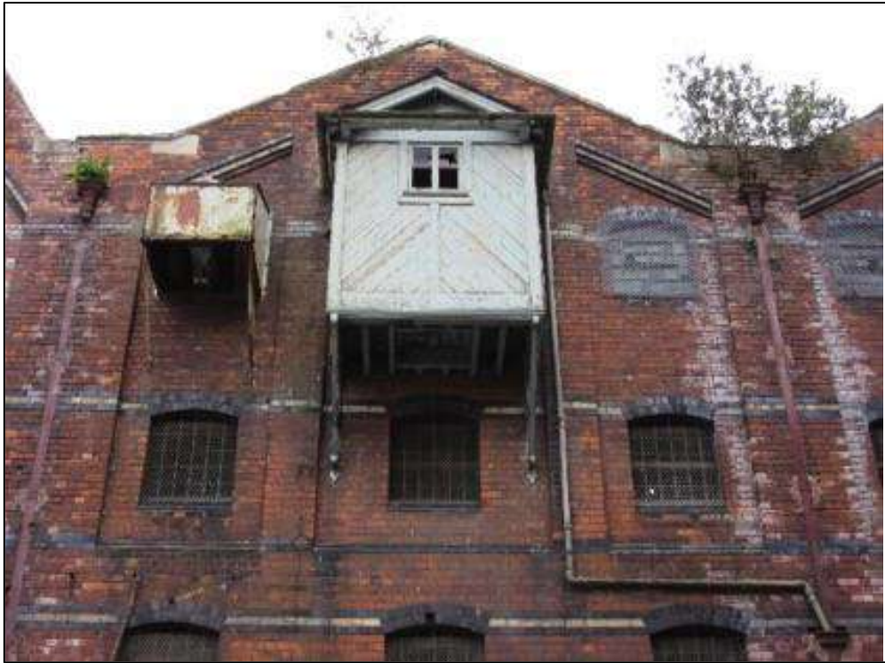
Fig.25 detail of timber hoist structure, western elevation
