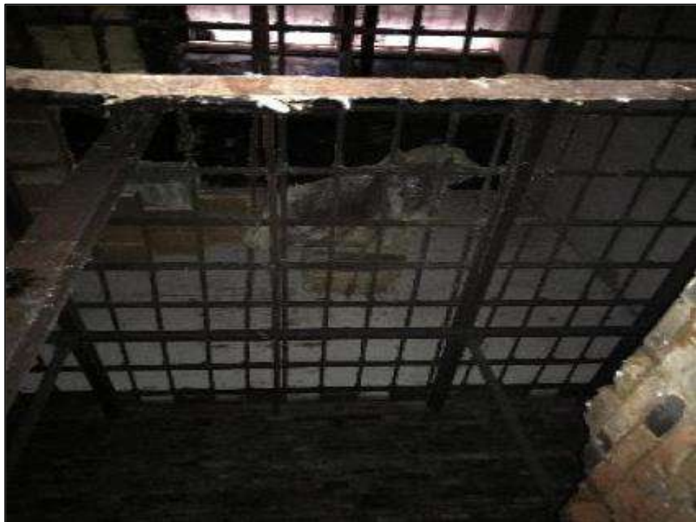
Fig.44 Detail of kiln drying floor, steel grid upon which perforated tiles were placed
