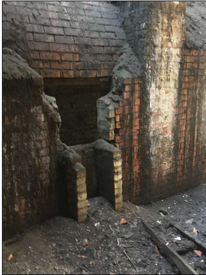
Fig.47 Detail of furnace opening viewed from the inside of the now lost furnace structure. The furnace would have been stoked from the exterior corridor
