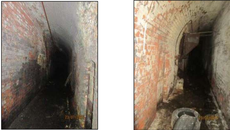
Fig. 43 Details of kiln furnace corridors with arch vaulting
