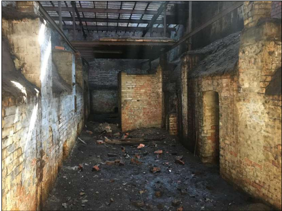
Fig.45 Detail of interior of east kiln showing profile of vaulted corridor running around the external walls, steel structure above and remains of furnace in the rectangular brick structure
