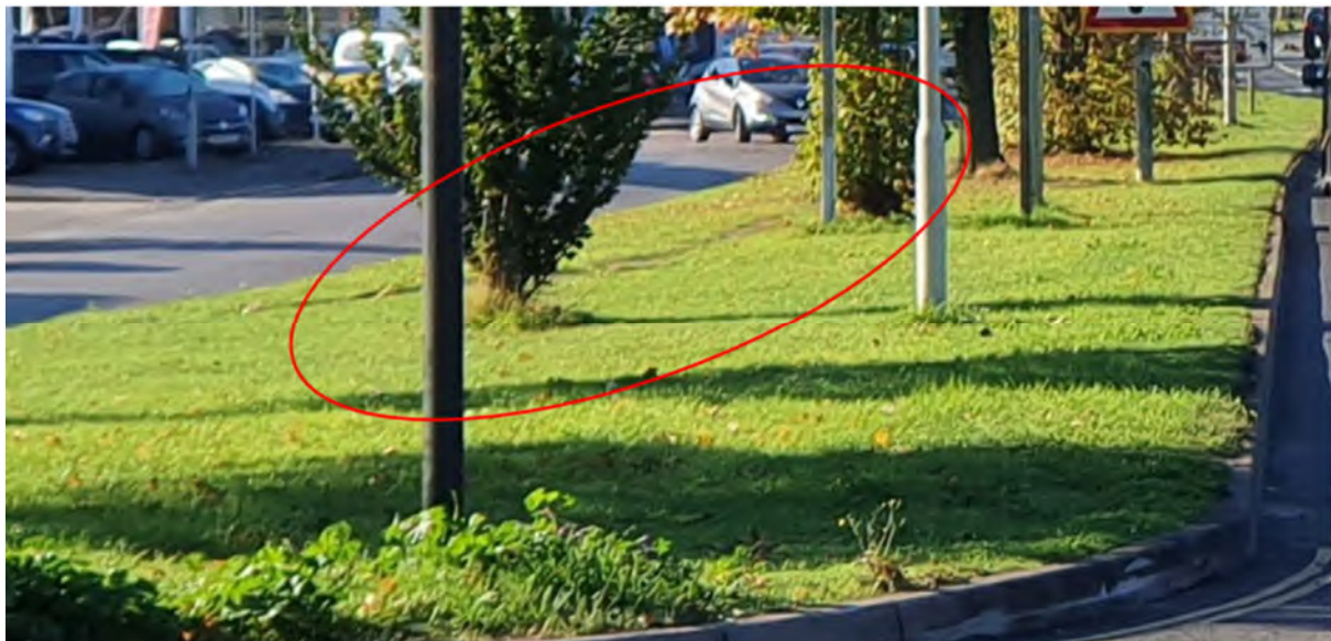
Figure 18: Lack of appropriate footway / cycleway on eastern side of Eastern Avenue.
