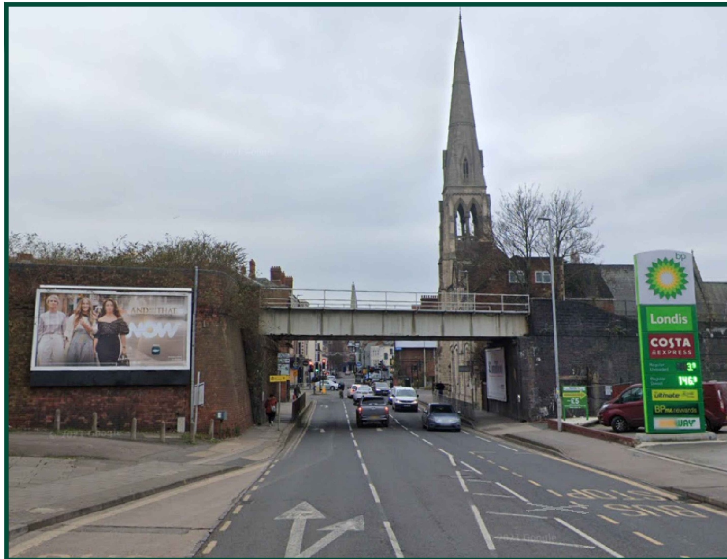
EXISTING SITE VIEW
