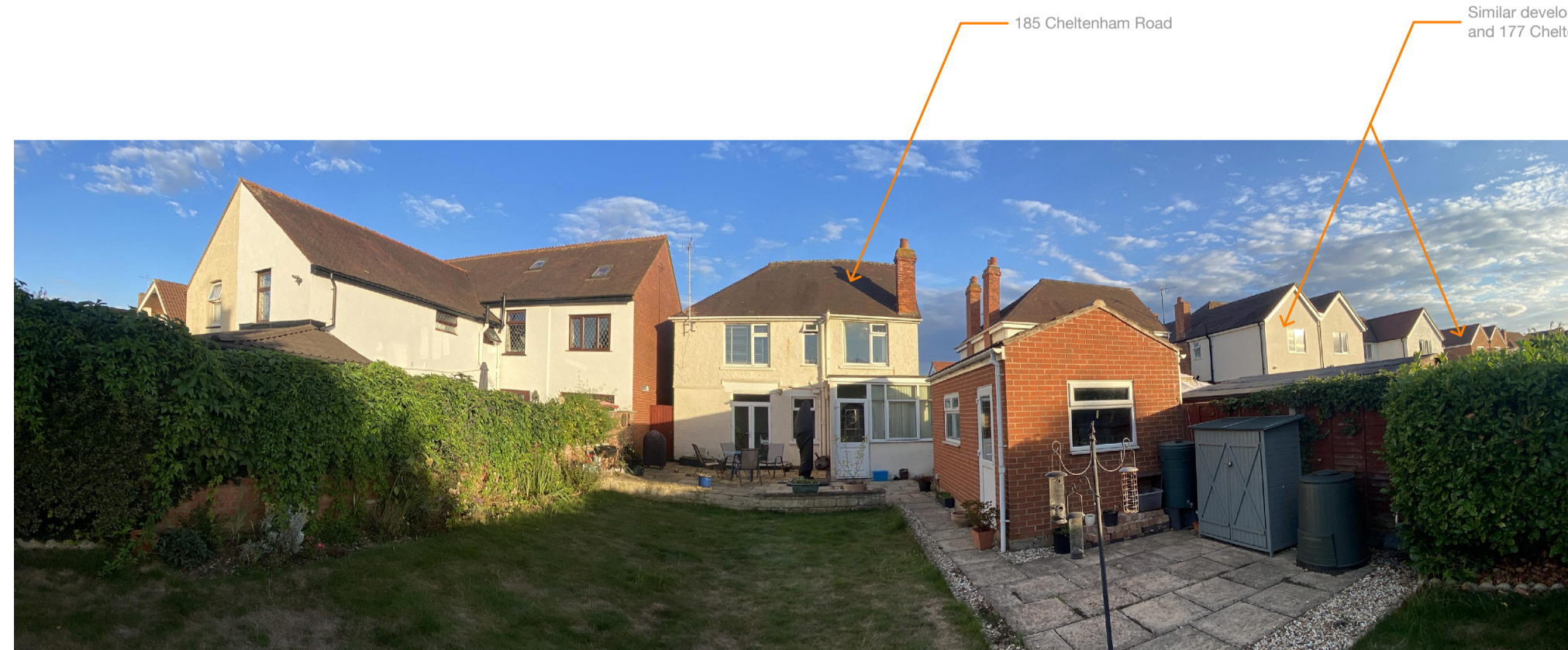
VIEW OF REAR ELEVATION
