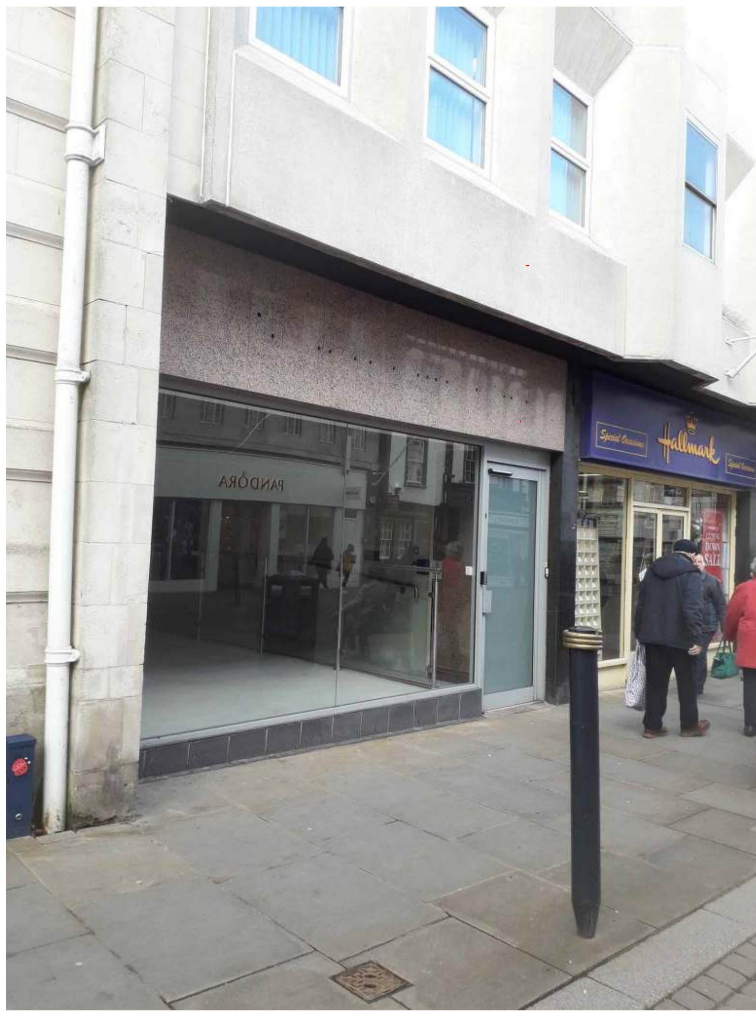
EXISTING PHOTO - SHOPFRONT
