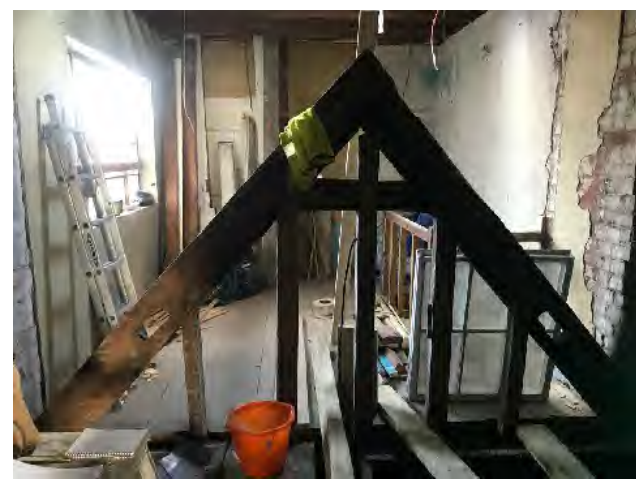
Existing Photo of Truss
