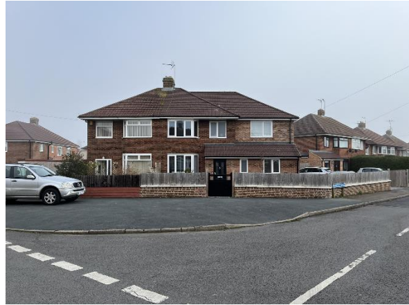
Front - from road junction.
