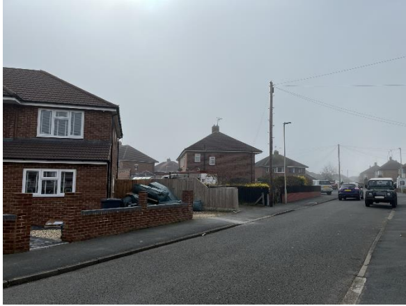
Towards side gable of no. 26.
