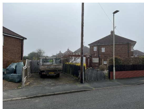
Side gable of no. 26 and sub station access.
