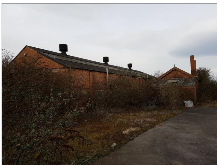
Photo 1: Example of the condition of buildings on Site.
