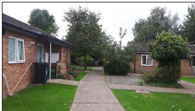
Photo 1: Buildings and hardstanding within the Site.
