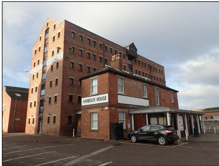
Photo 1: Buildings A and B.
