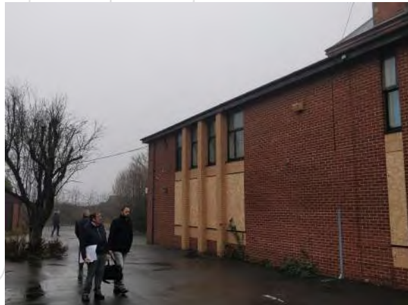
Side Extension and parking area viewed from site entrance.
