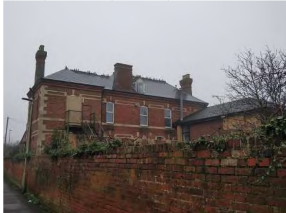
Rear of 18 Denmark Road viewed from Posy Lane.
