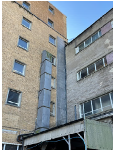
Photograph 4 - Boarding on the main building facing the courtyard
