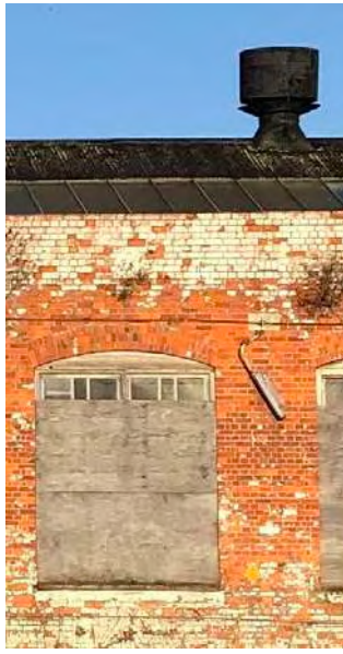
Local existing rail depot on site with worn painted red brick, brick lintels, metal roof and chimneys.
