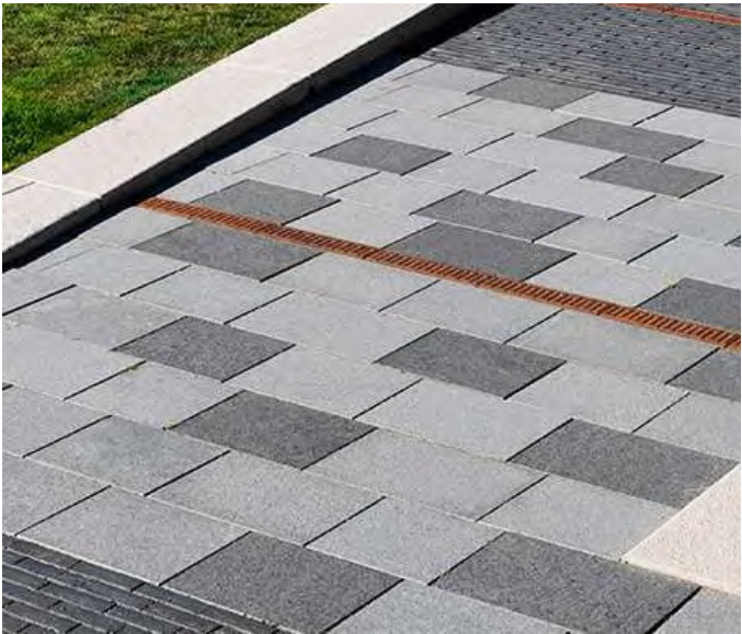
Permeable low carbon concrete paving
