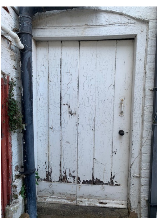
EXISTING DOOR D01 TO BE REPLACED
