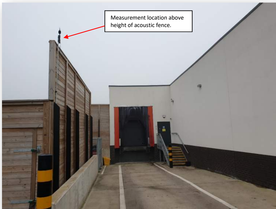
FIGURE 3: Baseline & delivery source noise measurement location.
