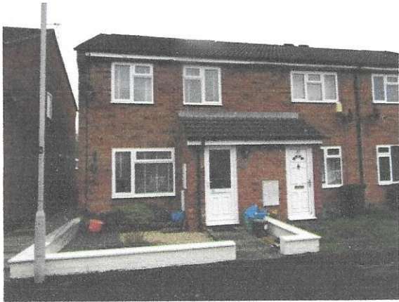
Application property and attached neighbour front view with landing window on detached neighbour side elevation
