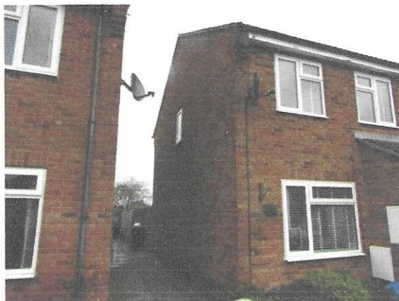
side elevation of application property showing stair landing window
