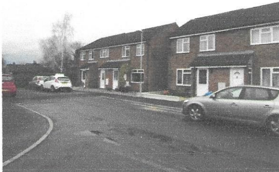
Front view looking towards detached neighbour
