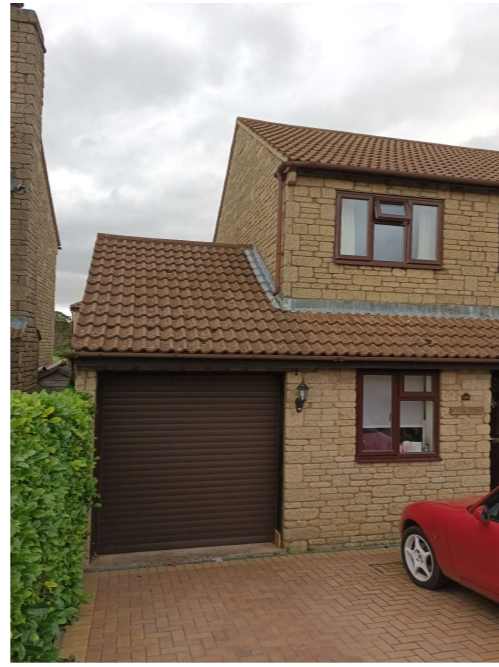
Garage to be converted
