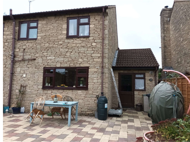
Rear View of Garage
