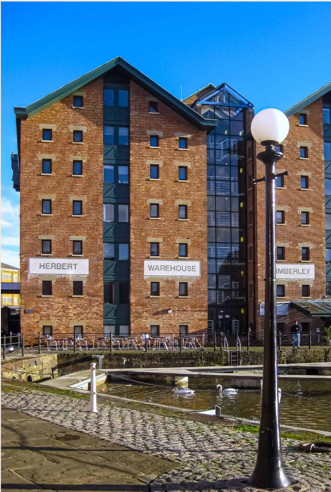
Fig 03.2 Herbert Warehouse, Gloucester Docks
