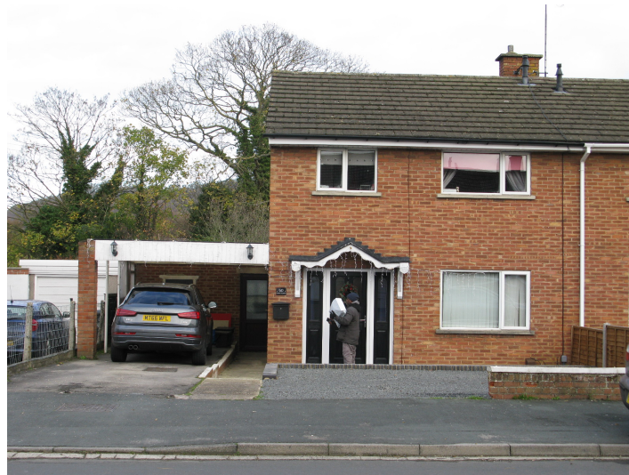
View of Southwest facing Front elevation with Carport
