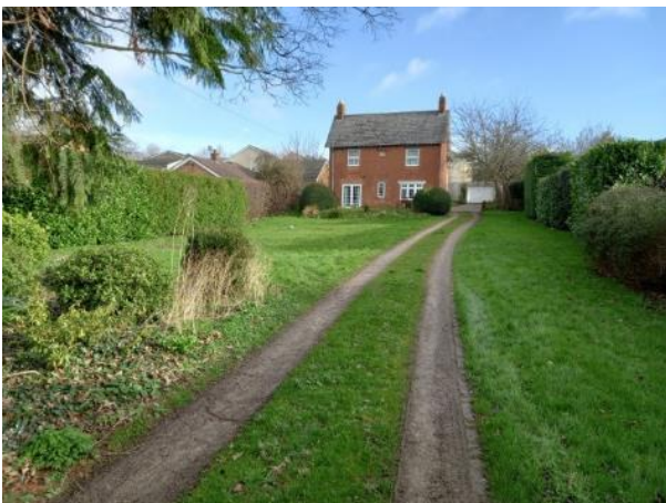
Plate 3.1: View of Paget Cottage from south-western garden boundary.
