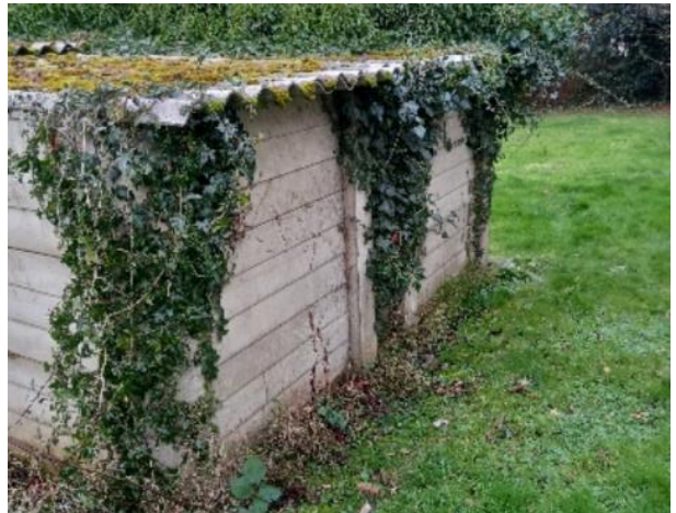
Plate 3.14: North side of garage.
