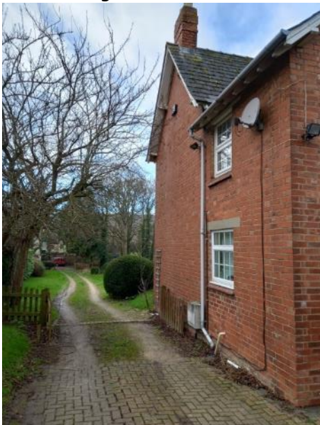
Plate 3.15: Paget Cottage, south-eastern elevation.
