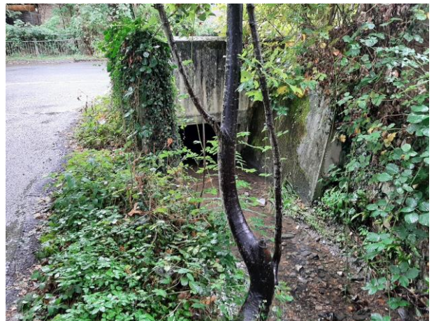
Photograph 5: Stream at culvert below road.
