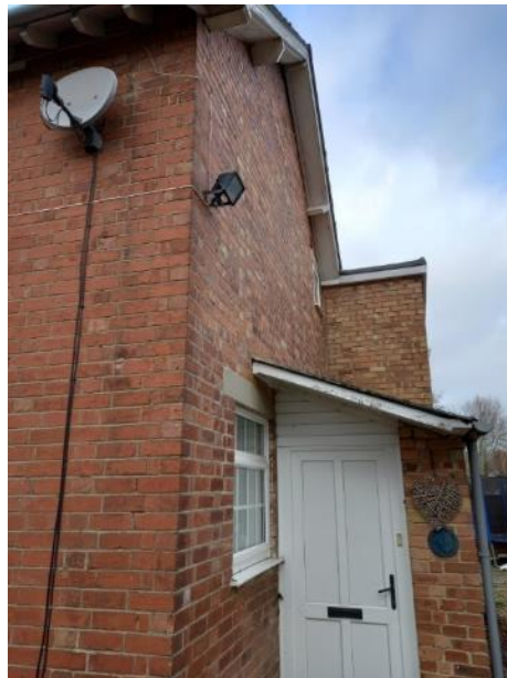
Plate 3.16: Paget Cottage, north elevation.
