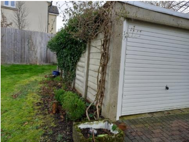
Plate 3.13: Concrete panel garage, view of western edge.
