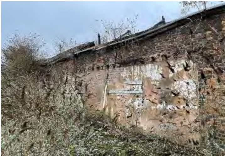
Plate 24: Evidence of former lean-to adjacent to Building 2.
