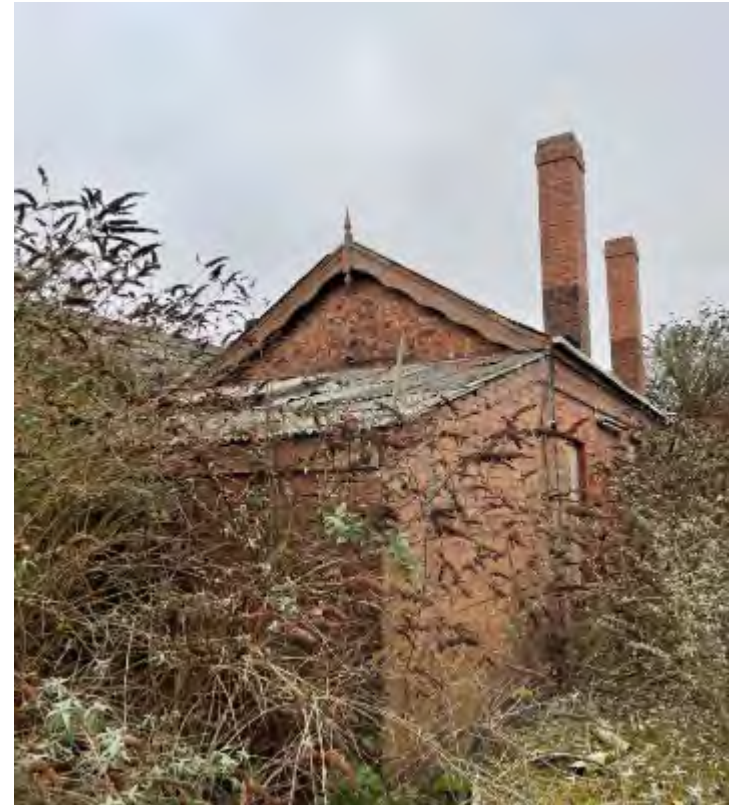
Plate 22: East end of Building 2 with modern extension, decorative bargeboards, finials and tall chimneys.
