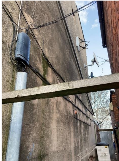
Figure 6 – Existing gable-end, 2 Oxford Street
