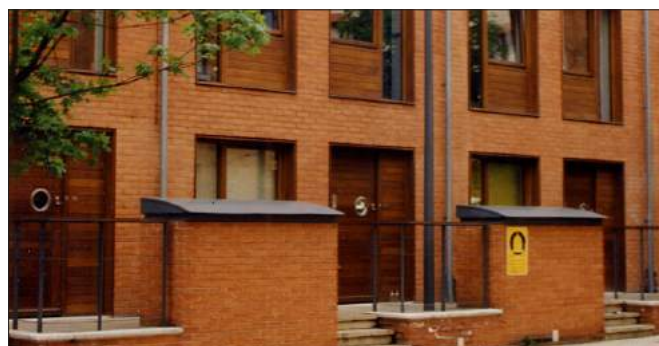
Fig 5.28: Bin storage positively designed into boundary treatment.
