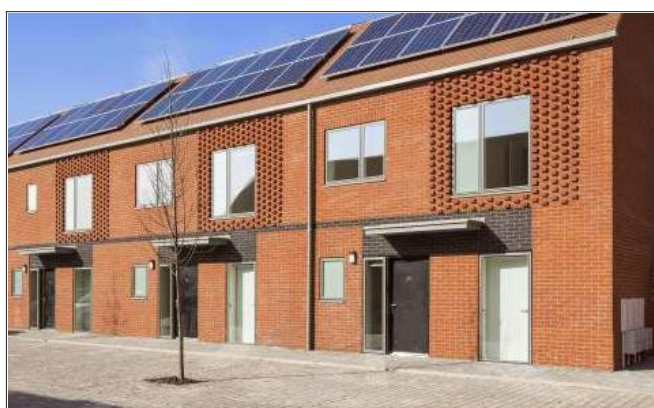
Fig 5.26: Textured brickwork provides robust three-dimensional interest that will stand the test of time
