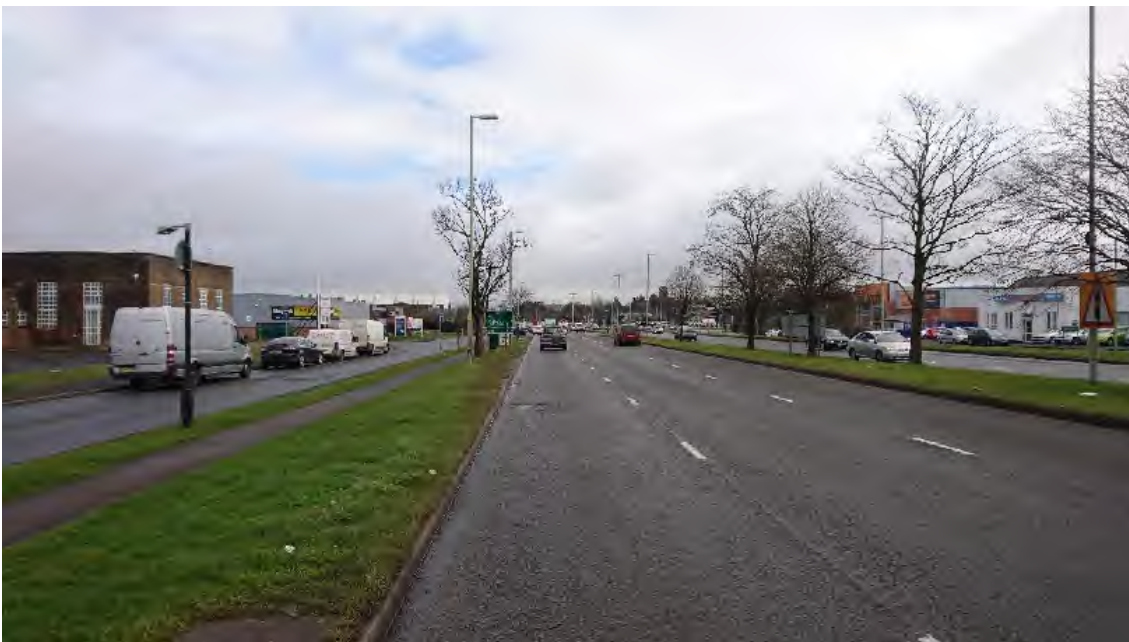
Figure 3: View looking towards existing Eastern Avenue / York Road junction.
